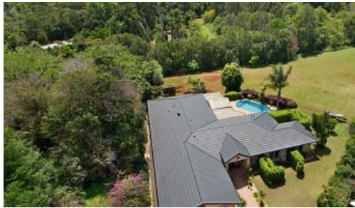
26 Kim Court, Alstonville
